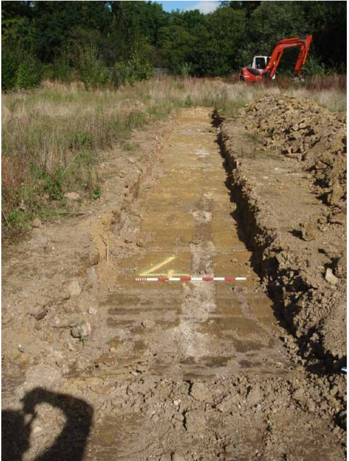
Plate 10. View of Trench 4
